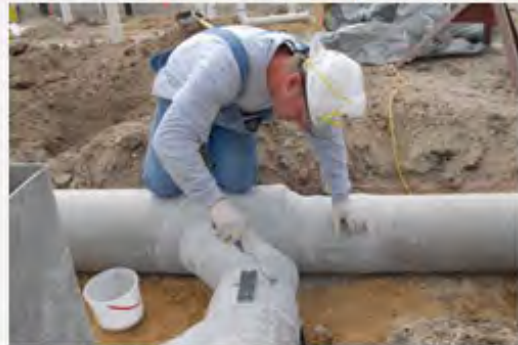
Installers prepare fiberglass and resin mix at jobsite. Installer places hot patch around UnderDuct.
