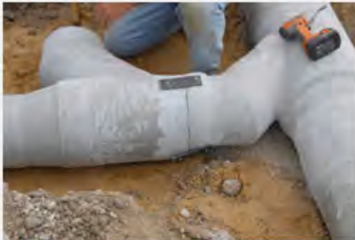
Edges to be joined are prepared and "roughed up." UnderDuct aligned and temporarily connected.
