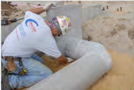
Installer welds strip to duct.
