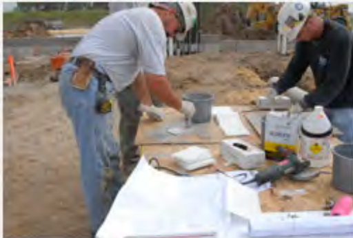
Installers prepare fiberglass and resin mix at jobsite. Installer places hot patch around UnderDuct.
