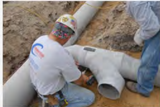
Edges to be joined are prepared and "roughed up." UnderDuct aligned and temporarily connected.
